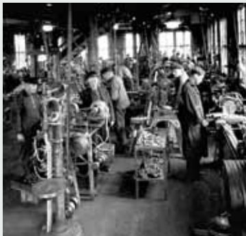
This image, from the early 1940s, shows the original workshop in Vaggeryd, Sweden. The current state-of-the-art operation at Vaggeryd is part of PMC Cylinders.
